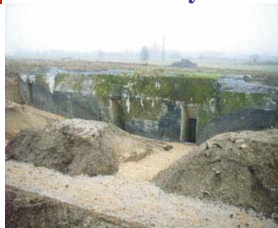
The Maisy Battery after 60 years underground
